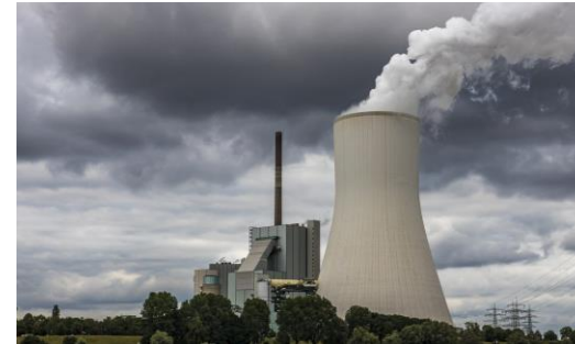
Power Generation Plant
