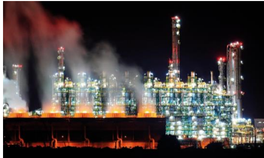
Downstream - Oil Refinery
